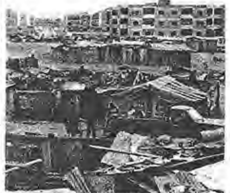
Last of Shanty dwellings in Detroit before their demolition
